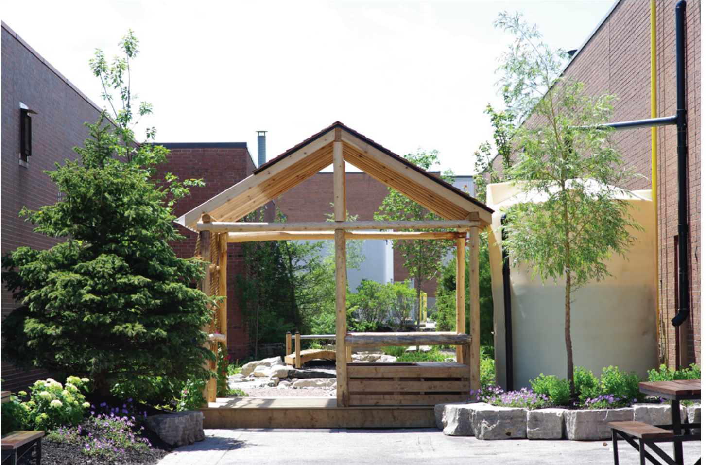
The Collective Stormwater Infrastructure Project at Calstone Inc., which features both a rainwater harvesting tank and retention pond seen above.
