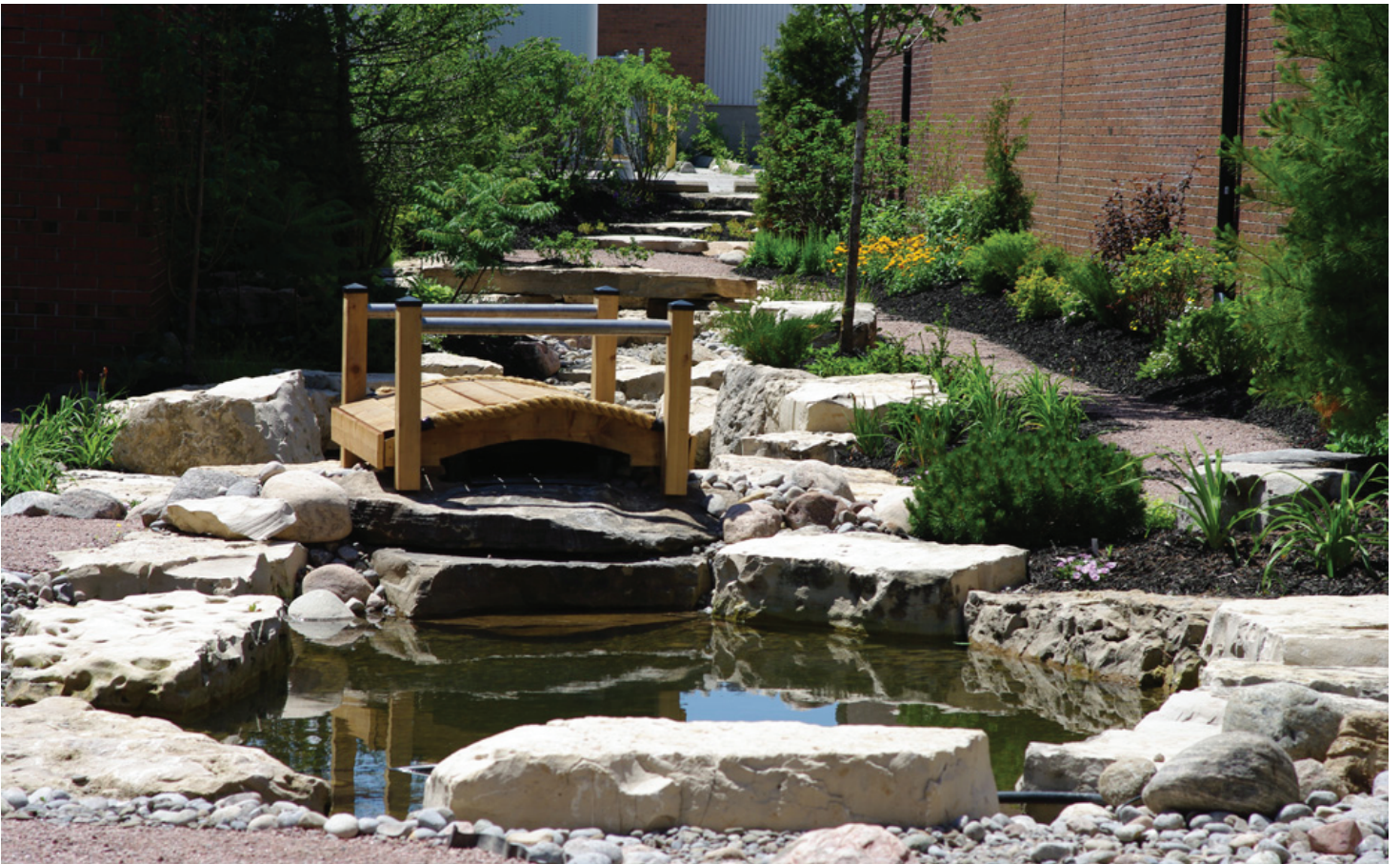
The series of stormwater retention and infiltration ponds at Calstone Inc.'s installation with Partners in Project Green.
