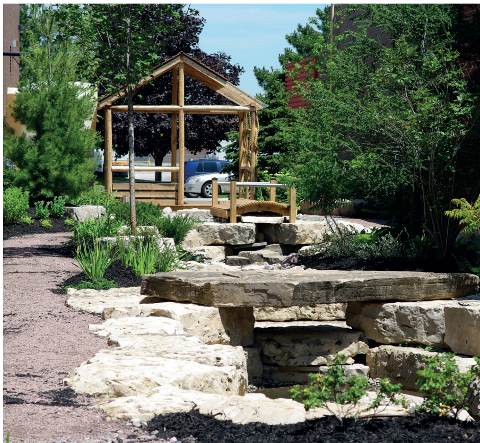
The interconnected stormwater detention and infiltration ponds on Calstone's property. The pond closest to the parking lot acts as spillover from Calstone's rainwater harvesting tank as well as a permanent, attractive water feature. Image by Partners in Project Green
